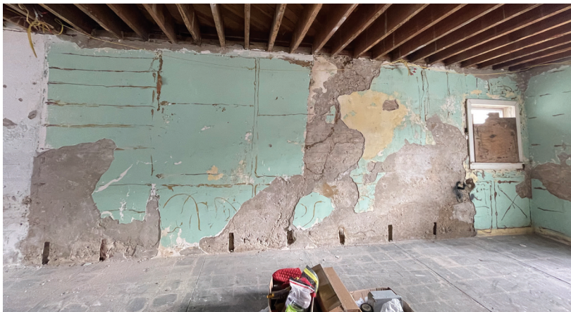
The extensive cleanup and restoration from 2022 to 2025 included major repairs in the basement (now Centennial Reception Hall) and the sanctuary, where the heart-pine floors and stained glass windows were restored to their former glory.
